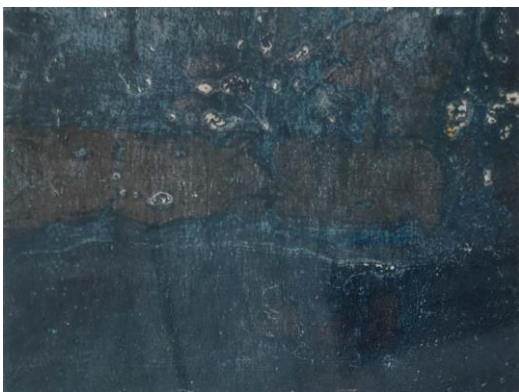
Figure 1-2 Rust Grade A
