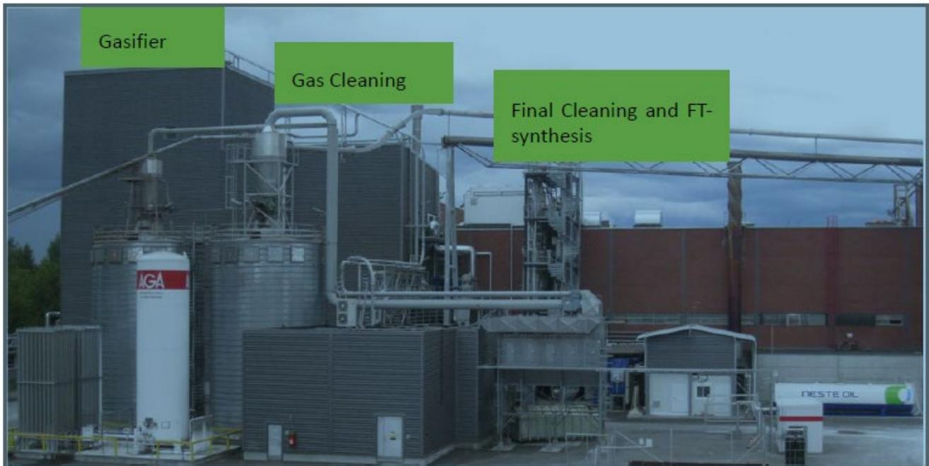
**Figure 12: NSE Biofuels Oy 12 MWth gasifier and 5 MWth slip stream gas clean up and FT synthesis plant, Varkus, Finland**
