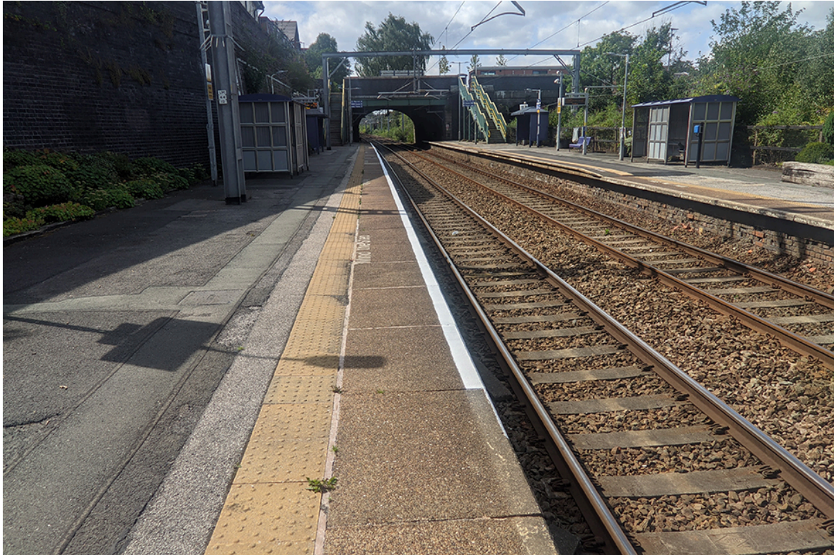
Eccles station platform 2 looking west, with bridge access in the distance
