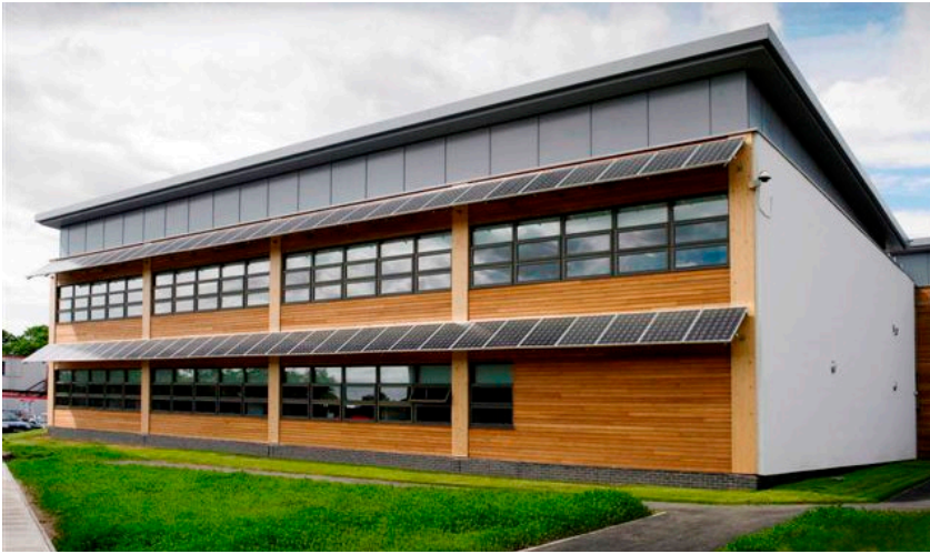
Figure 57: DEFRA office building in Alnwick (the UK's first zero carbon office) showing solar PV serving dual purpose as solar shading device
