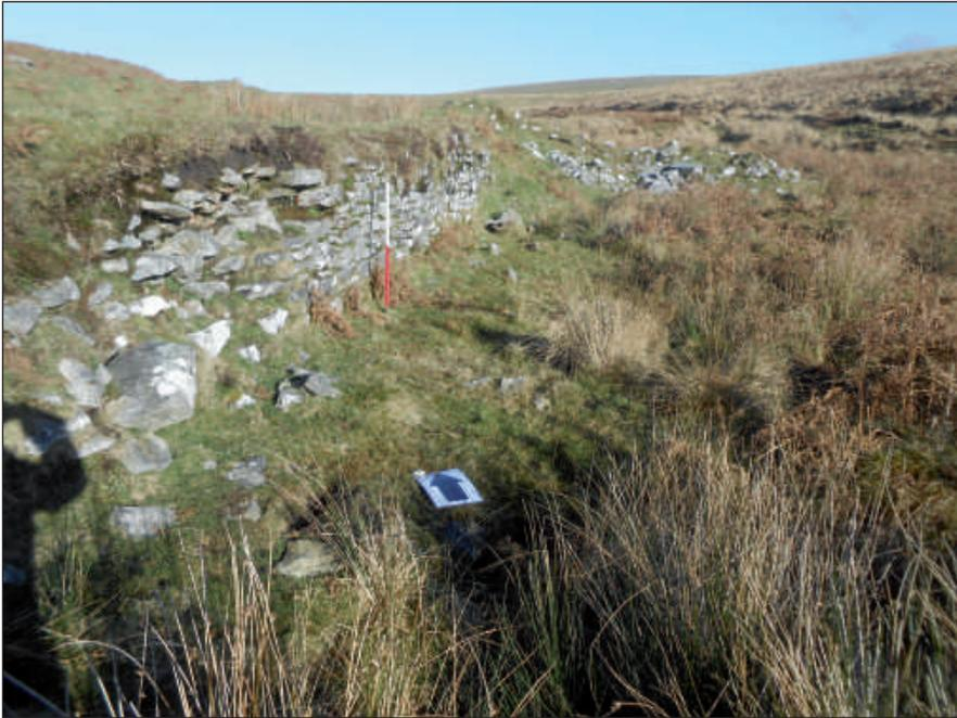
*Fig 11. 1318967 (SM No: 1021055) Stamping mill no 6 of Eylesbarrow Mine. The revetment wall of the tin dressing floor has suffered some collapse in recent years. Although beginning to stabilize.*
