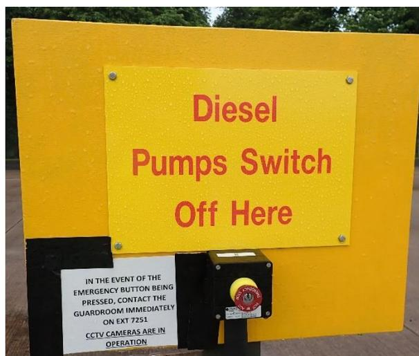
Figure 11 – Typical Dispenser Electrical Cut-Off at MTFI.
