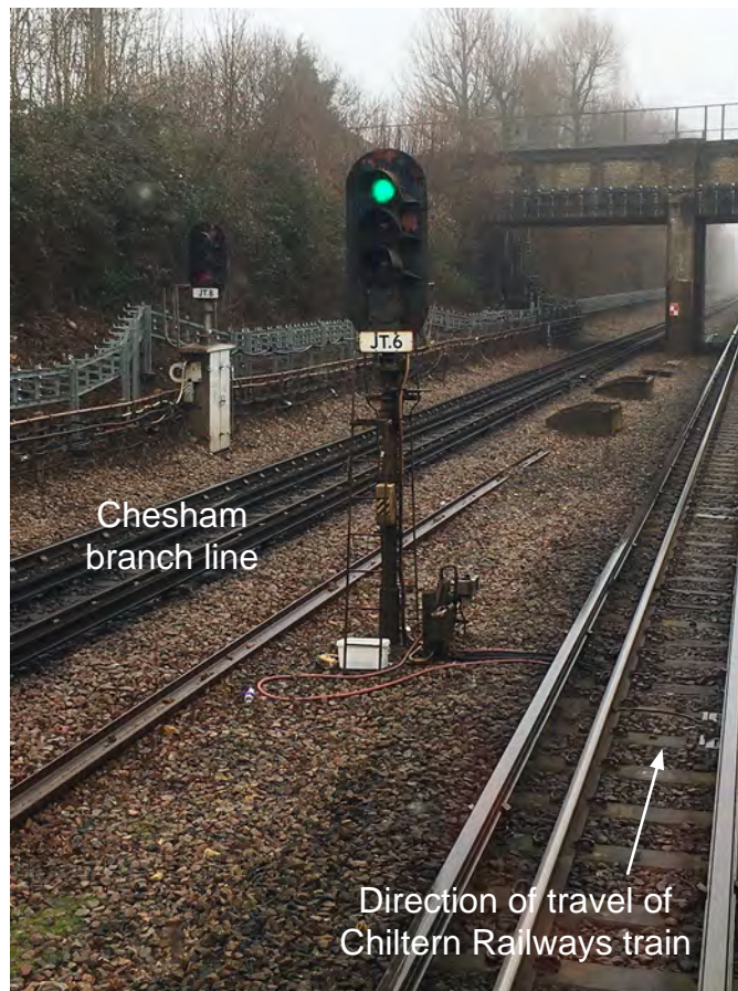
Figure 6: Signal JT6 (image courtesy of London Underground Ltd)
