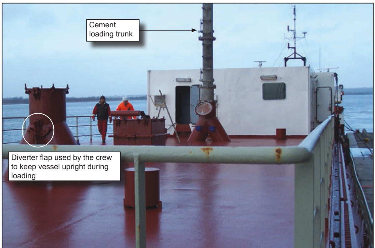
Figure 49: Cemfjord - cement loading cargo ports showing the diverter flap used by the crew to keep vessel upright during loading
