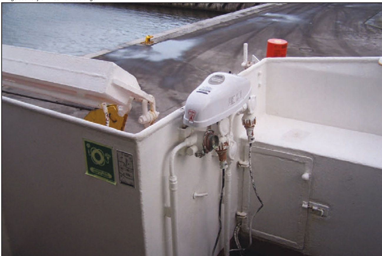
Figure 16: Cemfjord - EPIRB mounting arrangements on port bridge wing bulwark
