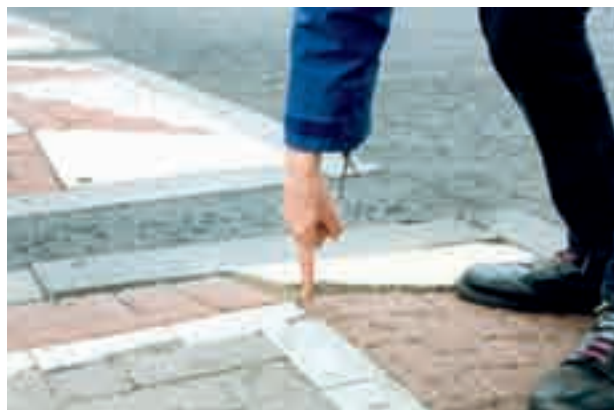
Fig. 2.8 Damage to a speed cushion
